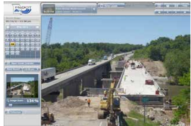
The fully constructed structure was slid into place.
