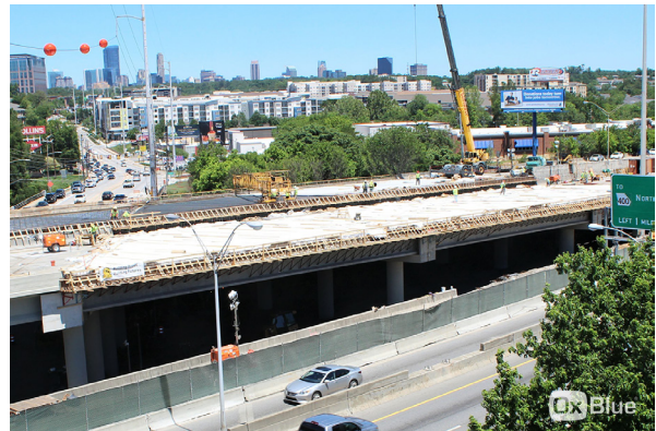
Image taken from OxBlue's fixed-position camera located at the I-85 construction site.
