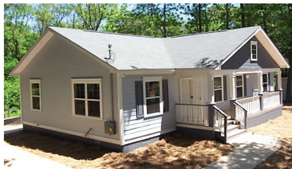
An OxBlue construction webcam captured a nine-day Habitat for Humanity Blitz Build in Atlanta.
